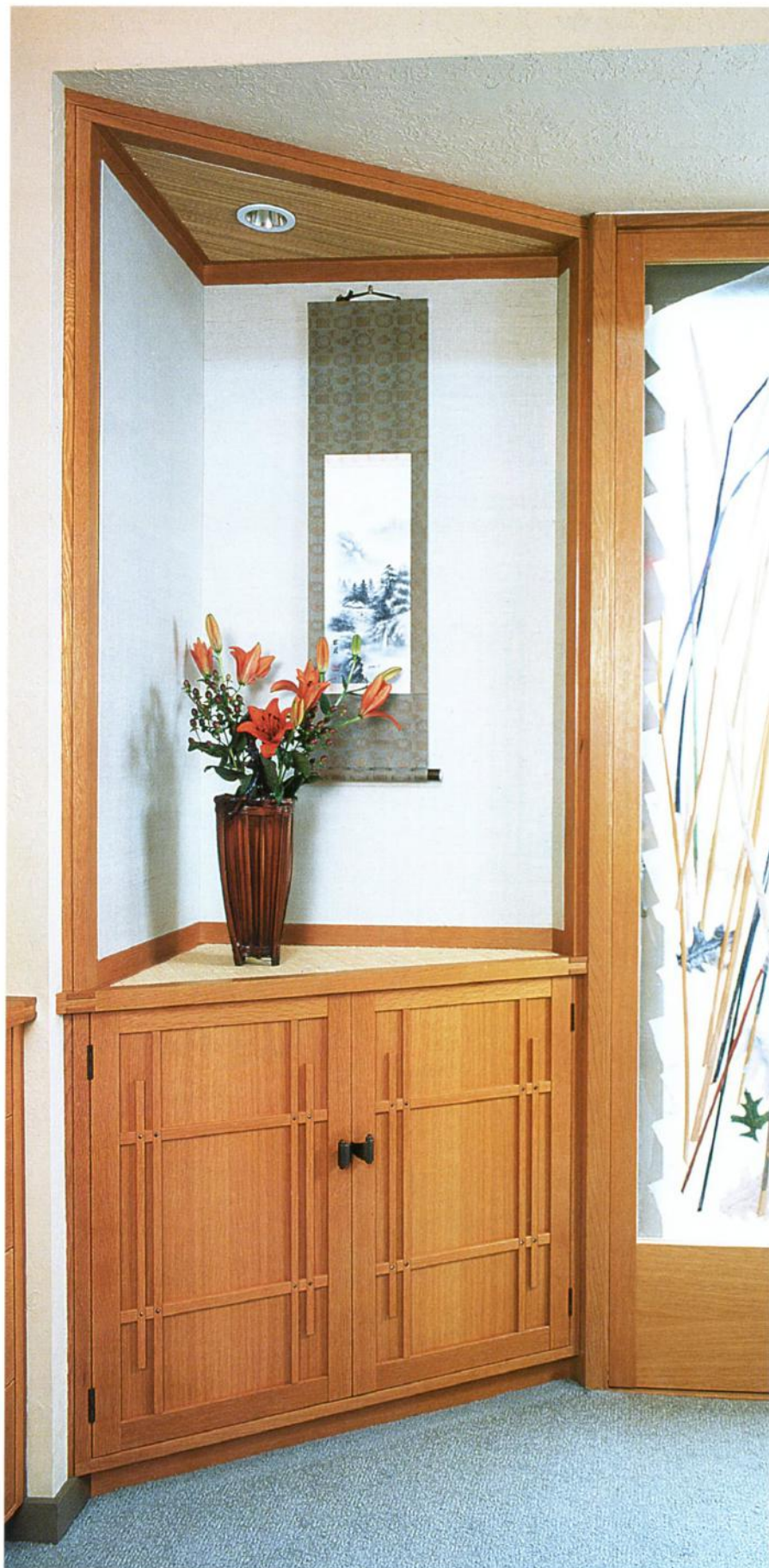
FABRIC ADDS TEXTURE. The top of the corner cabinet is covered in straw matting. The same material is also applied to the soffit.
